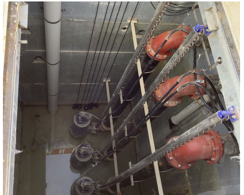
Legion Lift Station Replacement Project
