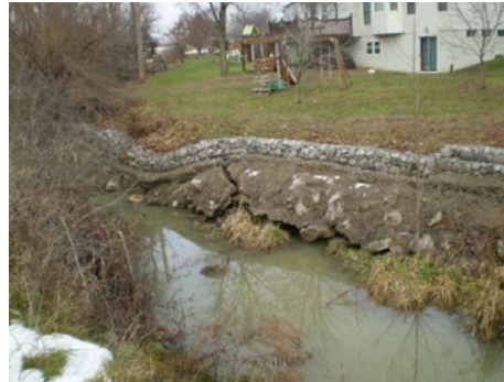
Hard armoring with concrete and gabion baskets on this bank is undercutting, causing more global failure.
