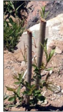
Cuttings from dormant riparian shrubs are planted deep enough in streambank soils to reach the dry season water table. These "live stakes" are used in a variety of bioengineering techniques. Stem nodes will take root. Nodes above the ground will leaf out.
