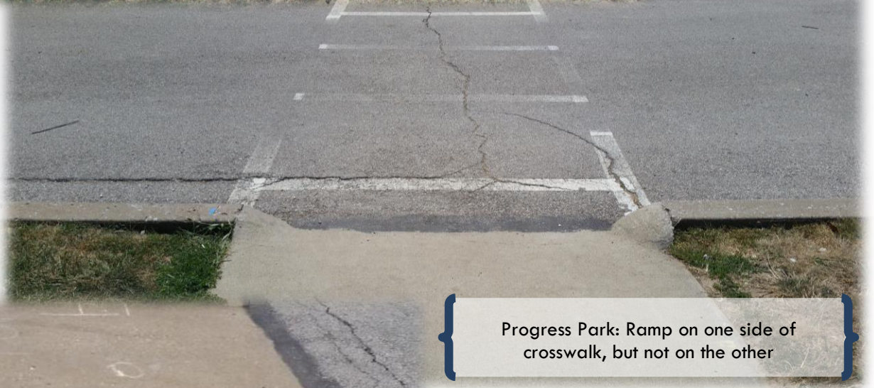
Ramp with no hand rail, "curb," and incorrect cross
