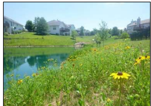
Common ground within the Huntsdale Subdivision, retrofit with native plants and rain gardens to soak up and filter stormwater.
